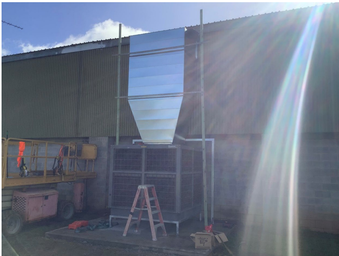
Figure 4: Gym Air conditioner upgrade
