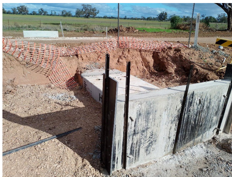
Figure 9: Culvert Extension Enmore Road
