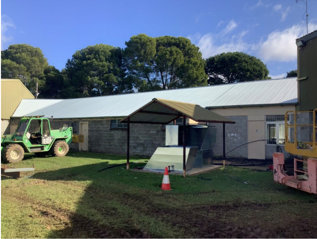
Figure 5: Roof improvements at the Narromine Sporting Complex
