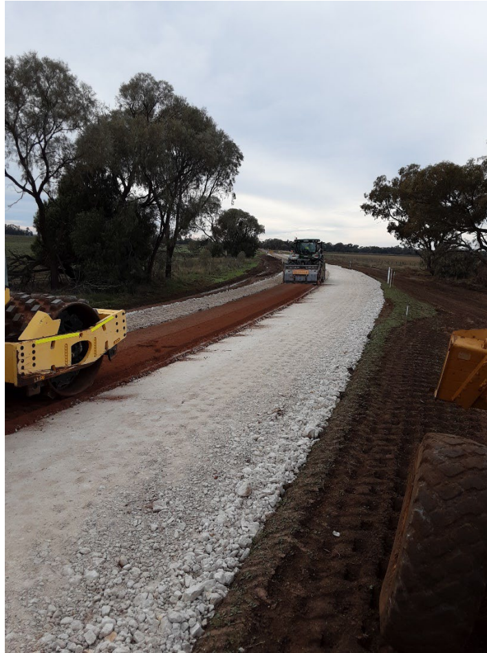
Figure 10: Construction works on Enmore Road
