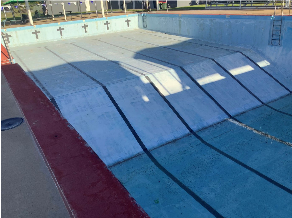
Figure 2: Current condition of Trangie pool.
