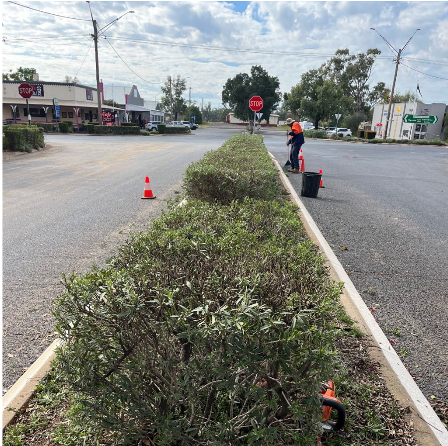
Figure 7: Works occurring in Trangie's Main Street
