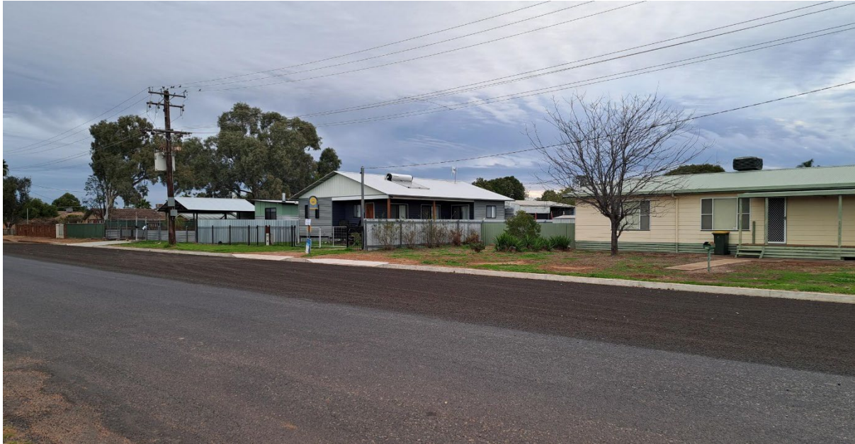
Figure 13: New kerb and gutter and wider sealed road on A'Beckett Street is looking fabulous
