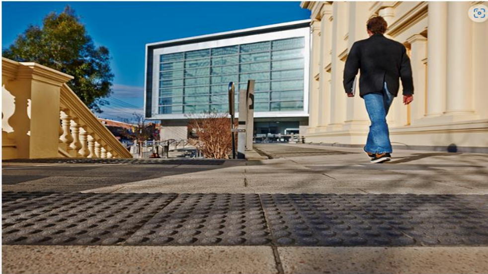
Figure 4.4 Tactile Ground Surface Indicators example (TGSIs)
