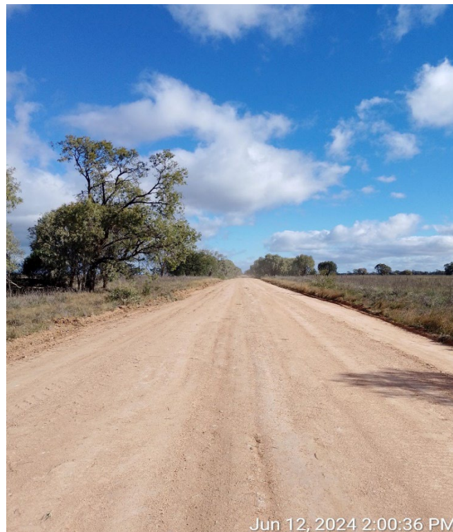
Figure 12: Jamea Road after maintenance upgrade
