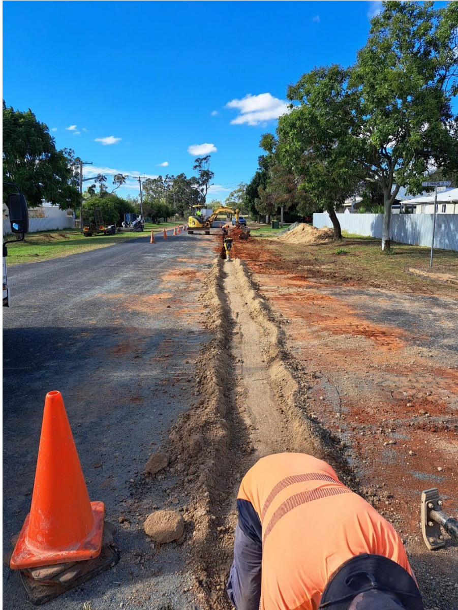
Figure 1: Installation of a new water main in Trangie
